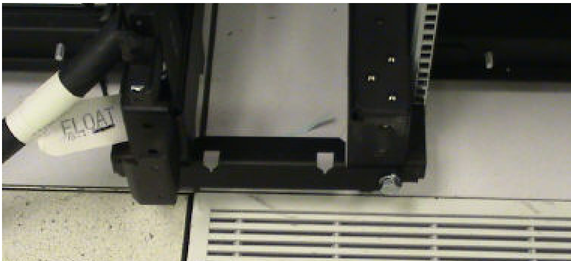
Figure 4-8 Rack Bonding Spacer – Bottom of Rack
