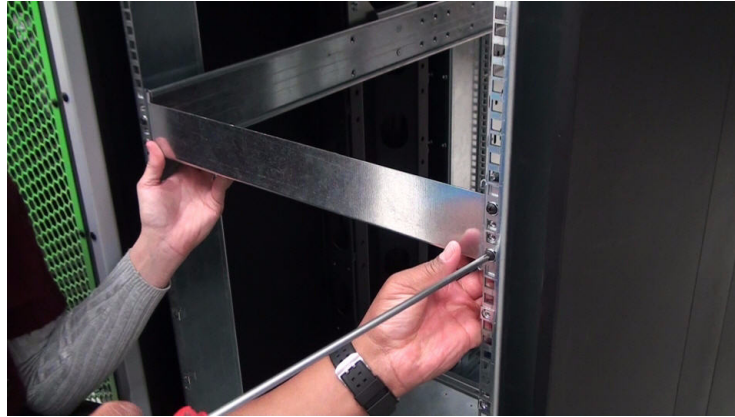
Figure 1-15 Adjustment Using the Alignment Tool
