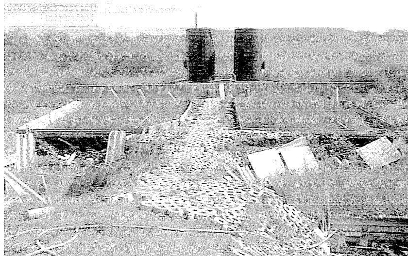
Figure A.30. A general view from the constructed wetlands (June 2002)
