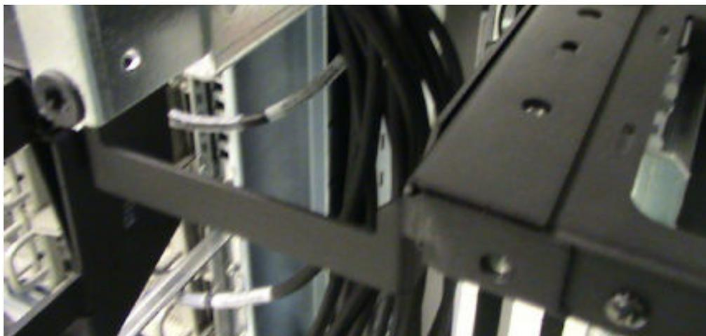
**Figure 4-7** Rack Bonding Spacer – Top of Rack
