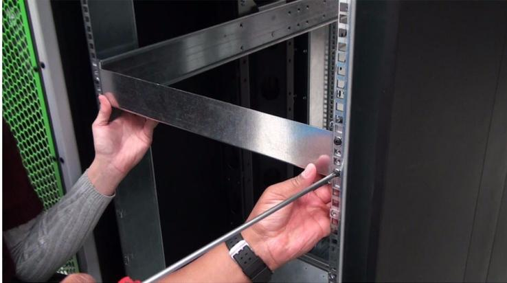
**Figure 1-14** Adjustment Using the Alignment Tool
