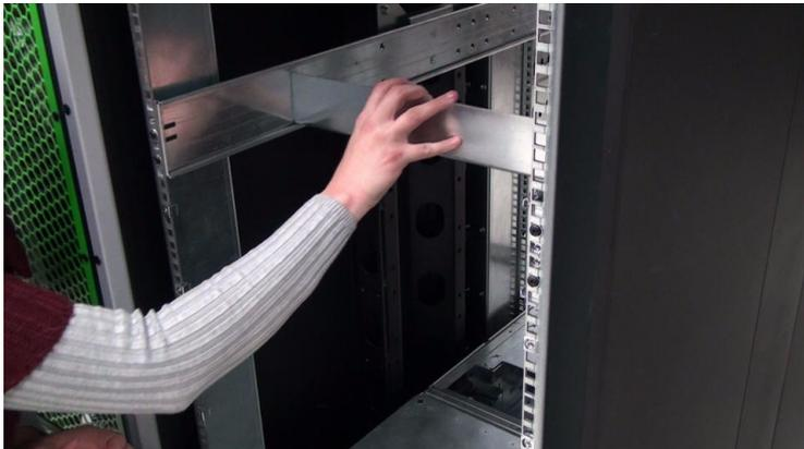
**Figure 1-15** Slide the Alignment Tool from Front to Back
