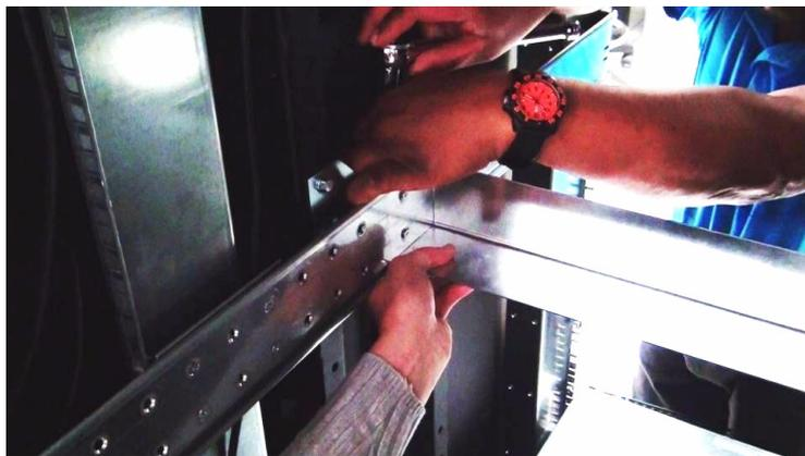
**Figure 1-13** Alignment with the D-Rack Stiffener Vertical Bolt
